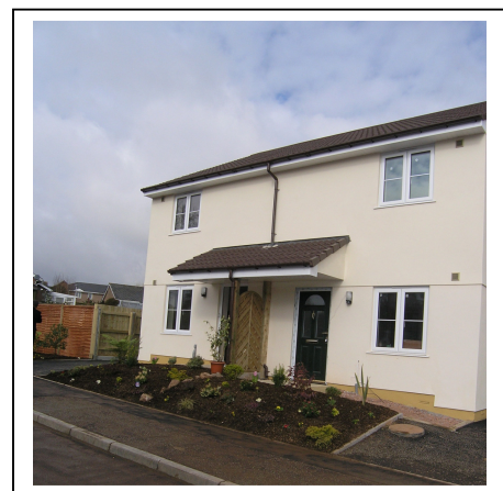
New housing association homes at Dunkeswell
